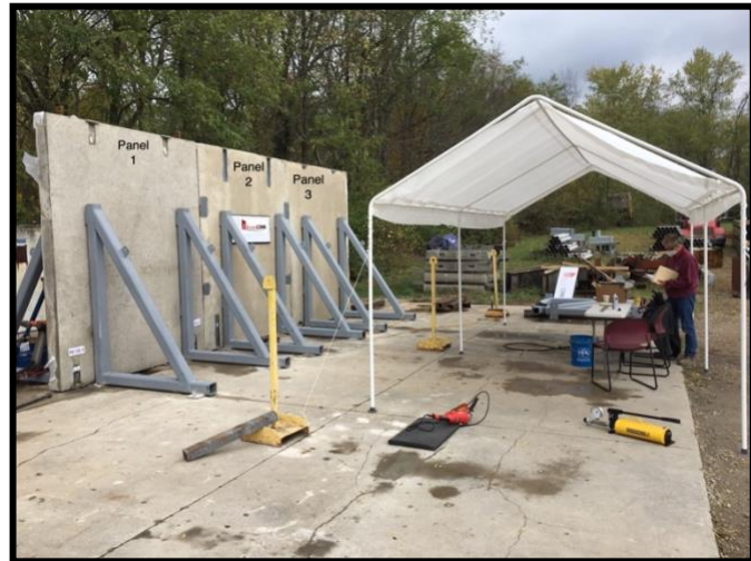
(b) Panels after installation of lateral braces
