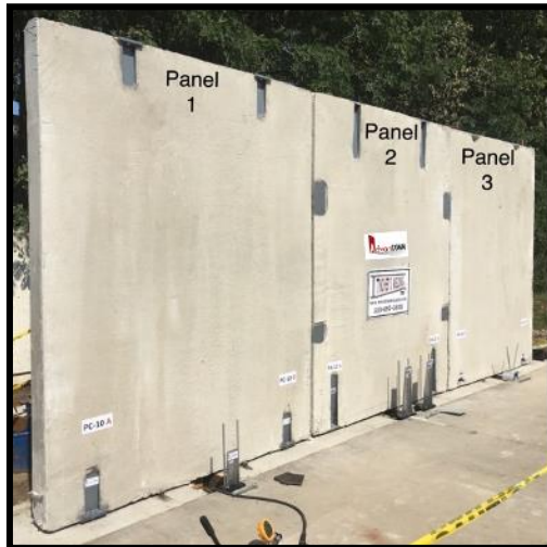
(a) Panels before bracing
