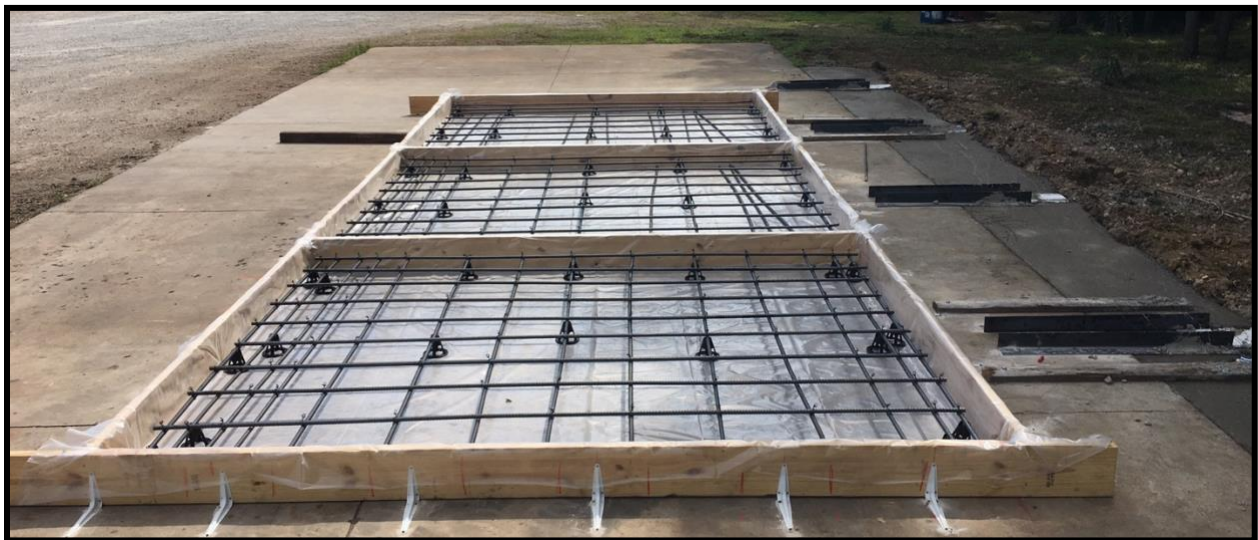
(b) Panels before concrete placement
