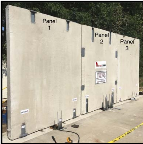
(a) Panels before bracing
