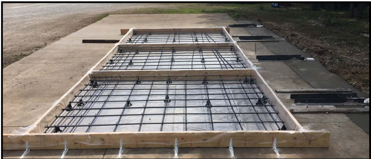
(b) Panels before concrete placement
